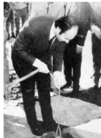
Mawlana Hazar Imam laying the foundation of a Jamatkhana in Khulna, India (1971).
