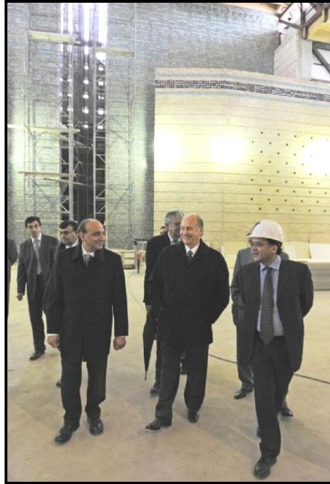
Mawlana Hazar Imam tours the prayer hall of the soon to be completed Ismaili Centre Dushanbe. He is accompanied by the building's Chief Architect and the Site Manager. Photo: The Ismaili Gary Otte
