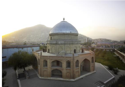
Timur Shah Mausoleum after restoration work by Aga Khan Trust for Culture. Photo: AKDN
