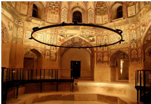
Conserved interior of the Great Hall of the Shahi Hammam, showing excavated cold pool, restored fresco work, a visitor walkway and lighting and illumination. Photo: AKDN
